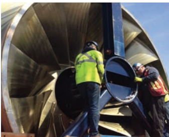
Churchill Falls, Canada 5,428 MW Refurbishment of ten large units and runner replacement
