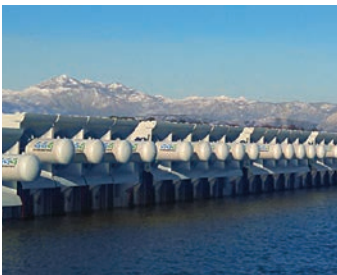
Ashta, Albania 24 MW + 45 MW 90 modules for the world's largest HYDROMATRIX* plant
