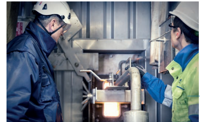
The liquor burners. The new boiler has cut mill emissions by 40-50%.
